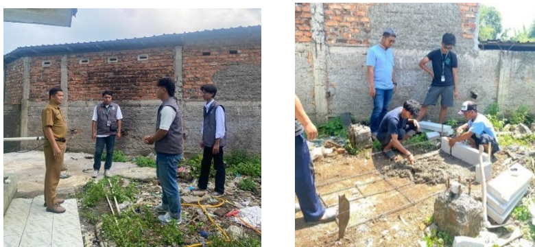
Figure 3 Socialization and Construction of Incinerators
