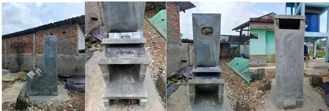
Figure 4 Results of Incinerator Technology Implementation
